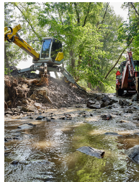
Hučava weir removal, Slovakia, 2021. © Rob Kleinjans
